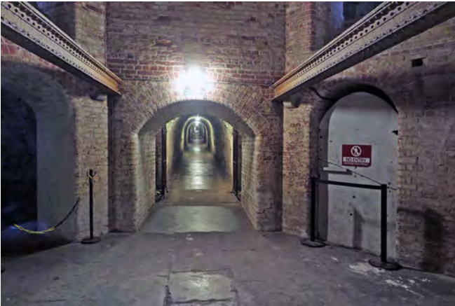
The Victorian tunnels under Fort Nelson, viewed from the counterscarp gallery. Temporary brickworks were established to provide the estimated 10 million bricks per fort required.
